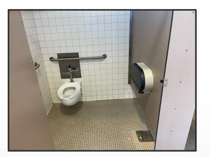
"Toilet paper dispensers shall be installed within reach, as shown in Fig. 29(b). Dispensers that control delivery, or that do not permit continuous paper flow, shall not be used. (4.17.3)"
